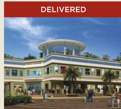
CITY SQUARE Commercial Complex at ACE City Sec-01, Gr. Noida (West)
