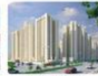
ATS ADVANTAGE PHASE II Gurgaon
