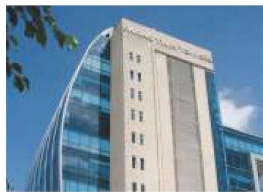
PARAS TWIN TOWERS
